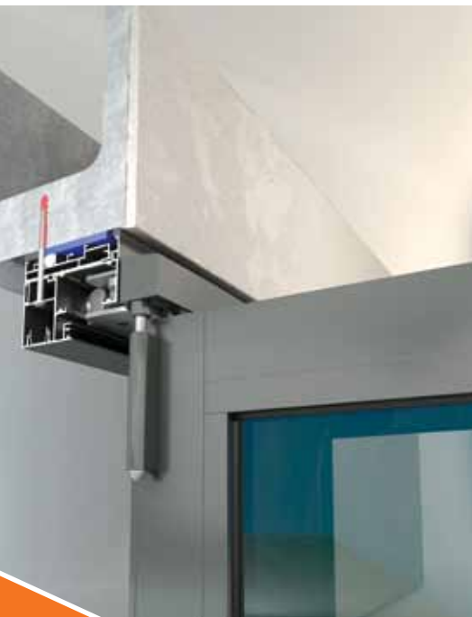
Inline™ Bifold Door head detail
